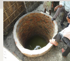
Pits smaller than required
