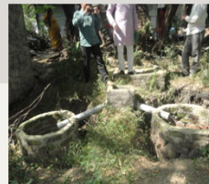
Pits smaller than required
